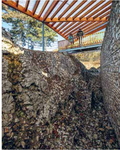
The new protective roof over the trench.
